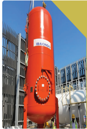
Surge Vessel Installations
