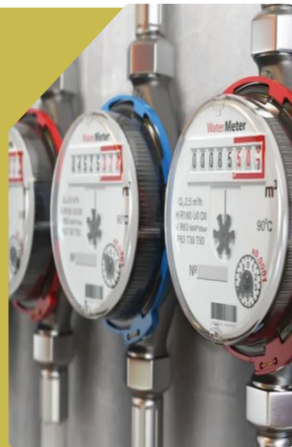
Water Meter Installation
