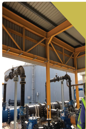
Midfield Bypass Line Installation
