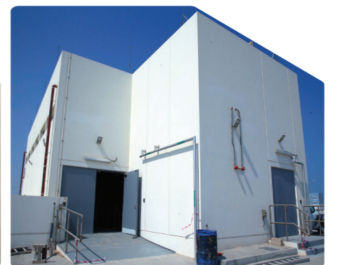
Cargo Terminal - HIA
