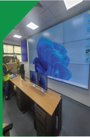
Vlideo Wall Screen Installation
